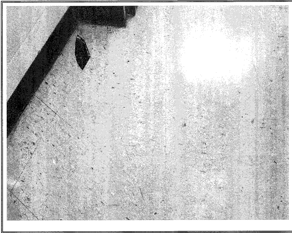
PHOTO 3: 12" Tan Floor Tile in Corridor at Room 103.
